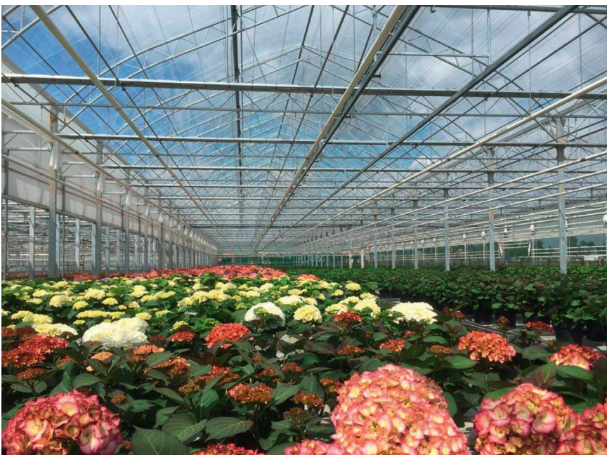
Fig. 3. ETFE greenhouse films are long-lasting and can promote plant growth. The greenhouse in the picture has a surface area of 5000 m 2 and has been covered with a single-layer F-Clean film
